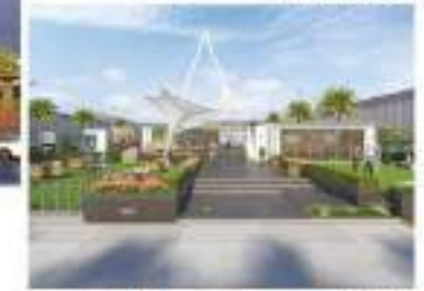
Indraprasth Industrial & Logistics Hub (Warehouse)
