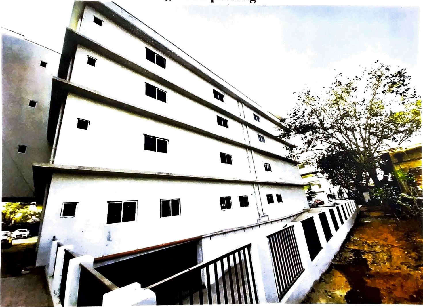
Image 2: Side view of the building and ramp for underground parking
